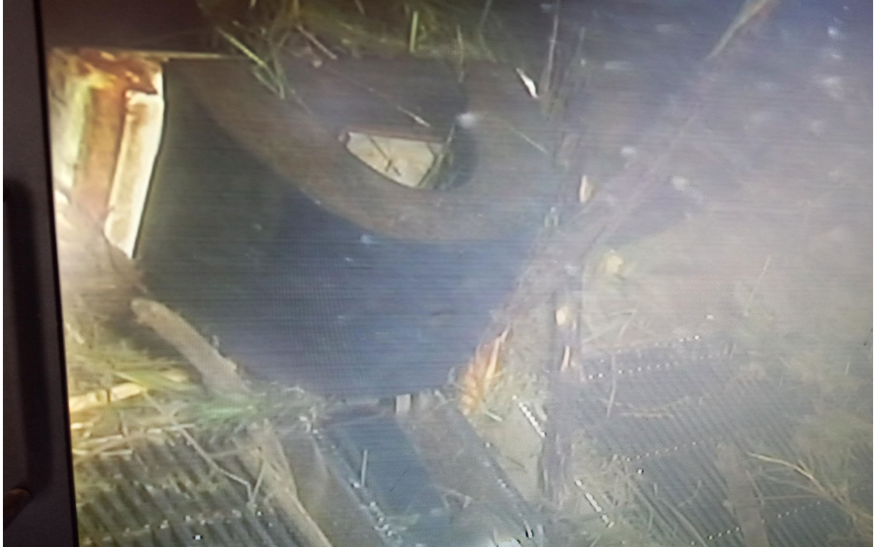
Photo 4: Debris on the top bumper on the ESBS in 1A slot.
