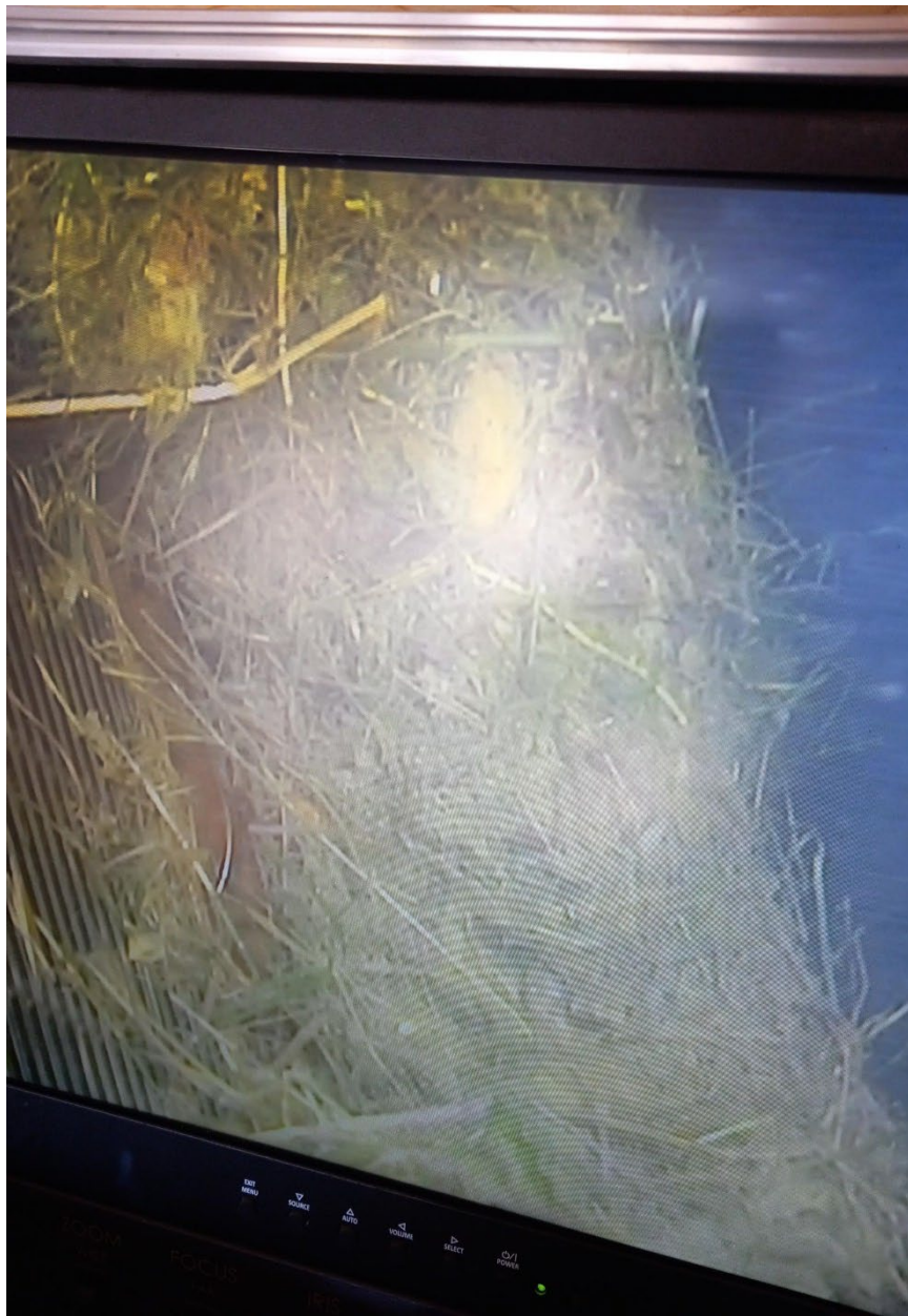
Photo 6: Debris wad on the ESBS in 1B slot.
