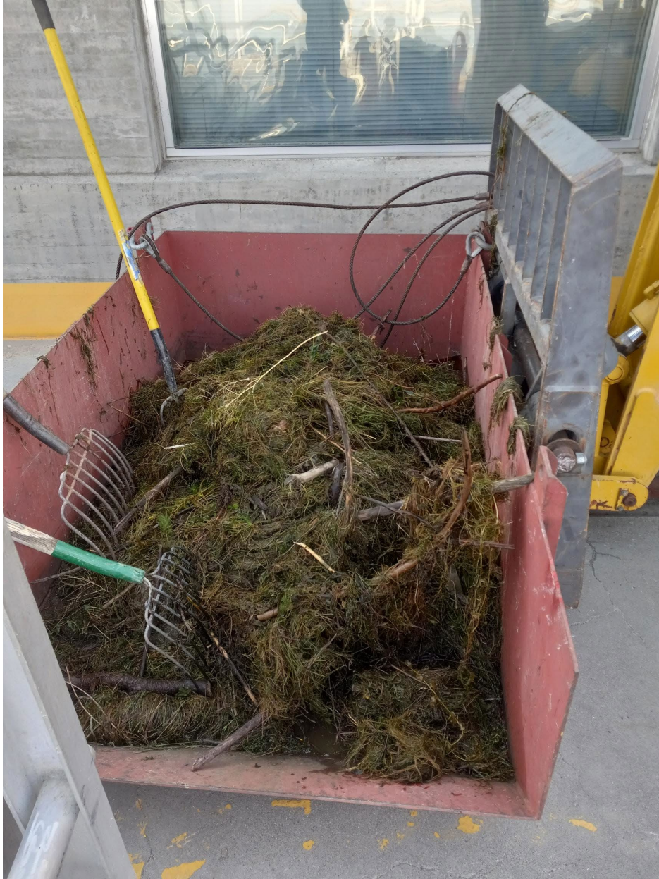
Photo 7: Debris removed from the two ESBS's (mostly the screen in 1A slot).
